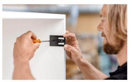
Our assembly devices assist you in processes such as positioning and fastening the AVENTOS lift mechanism to the cabinet. Optimal alignment ensures that the fittings function perfectly, making opening and closing a pleasant experience for your customers.
